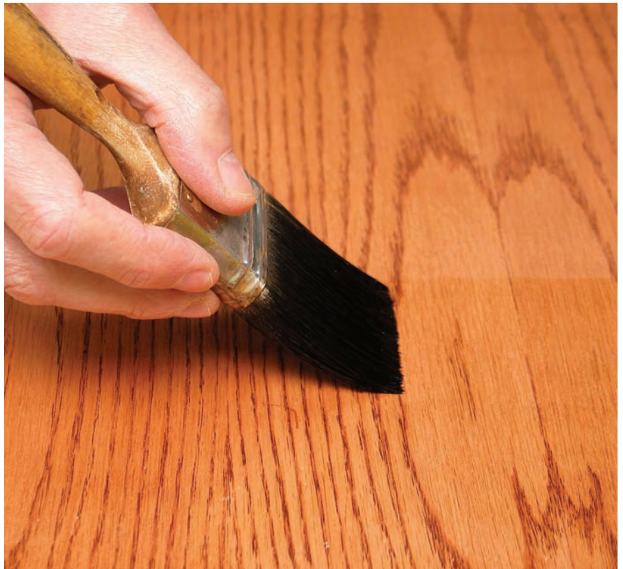
No advantage. It's not necessary to brush across the grain, as I'm demonstrating here, to work the finish into the wood. The finish penetrates perfectly well by capillary action no matter how it is applied.
